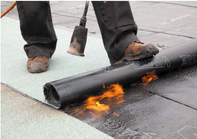
The polymer bitumen sheeting VEDATOP DUO reliably protects the roof against weather-related damage and ensures an attractive visual effect due to the dolomite grey sprinkling. Source: Vedag GmbH
