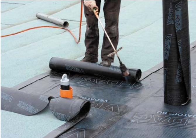
Incorporation of details into the double-layer waterproofing is enabled without problems. Source: Vedag GmbH
