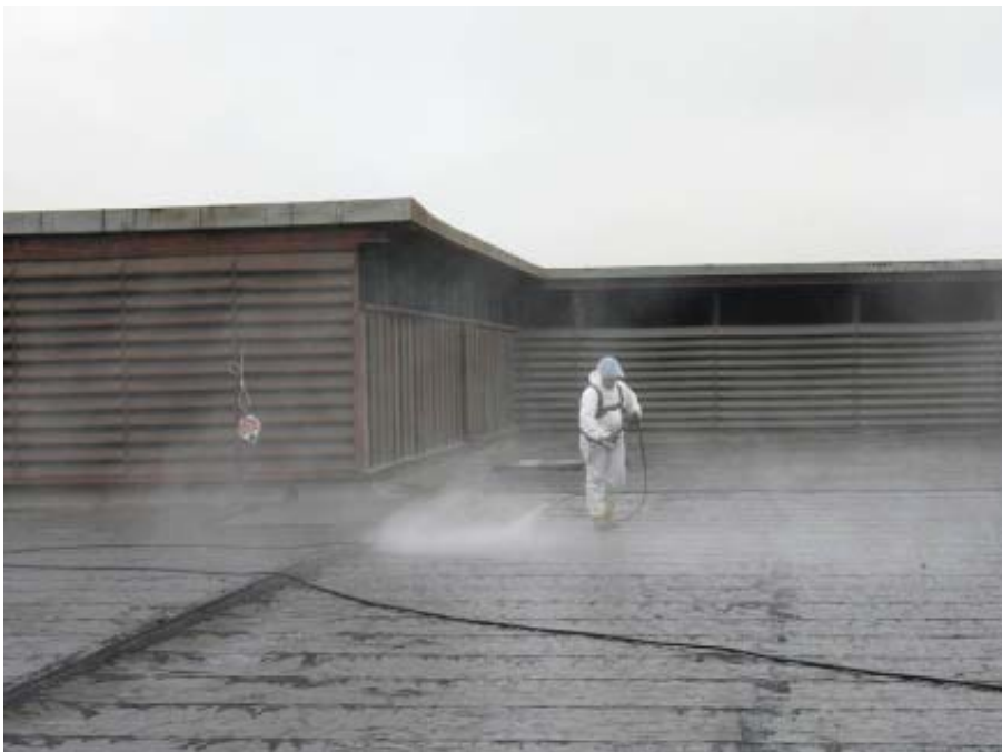
The heavily encrusted old roof had to be intensively cleaned beforehand.
