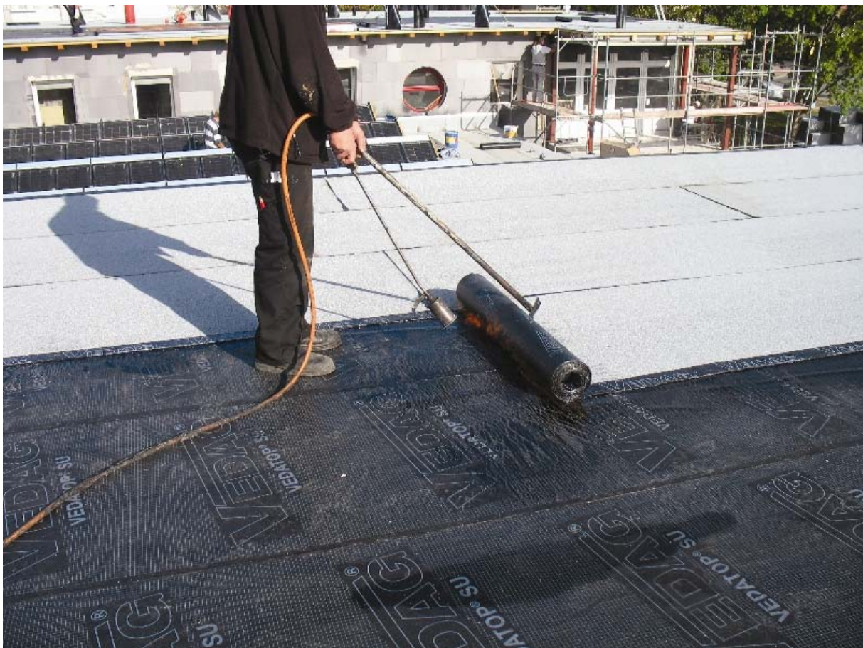
The dolomite-grey polymer bitumen sheeting VEDATOP DUO is welded on as a top layer. Photo: VEDAG
